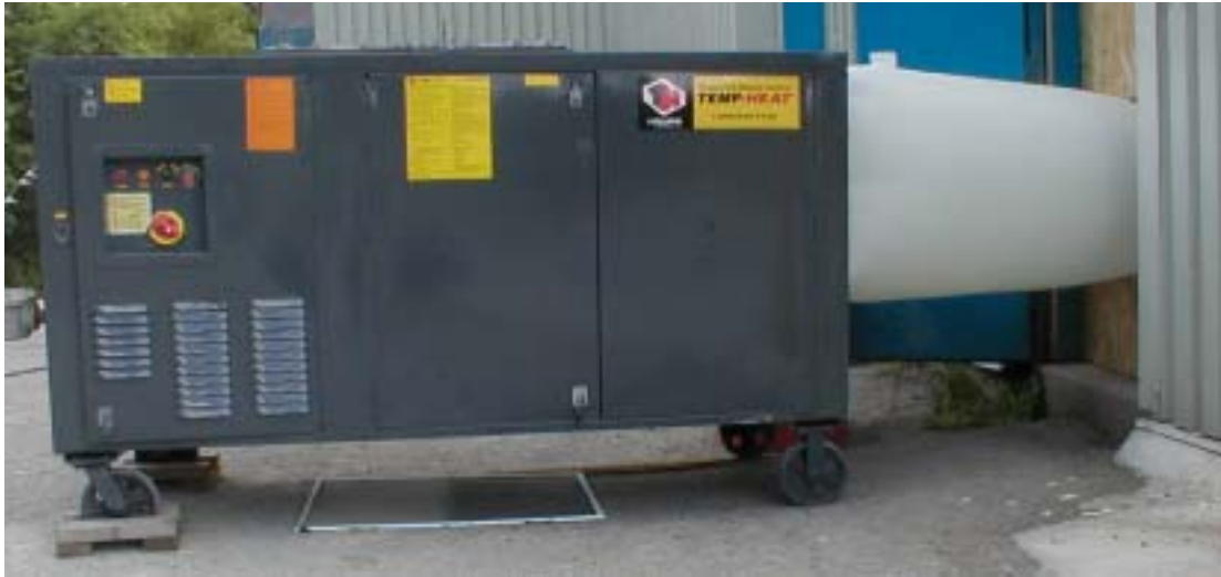
Figure 1. Propane-fired heater (Temp-Air) heating Mill 1. The door has been sealed with plywood, and a flexible cloth duct delivers heated air through a hole cut in the plywood.
