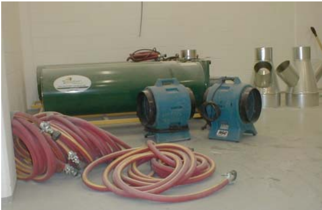
Figure 2. Low-pressure steam heaters waiting to be attached to steam. The metal ducts (on right) were attached to the end of the heaters, and flexible wire and plastic ducts were attached to distribute the heat. A total of 10 blue fans were placed throughout the building, in addition to one Roo-Can fan.
