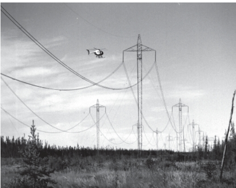
Fig. 3. Sample Steel Towers
