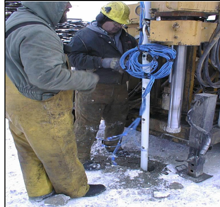
Fig 5. Installation of Thermocouple strings
