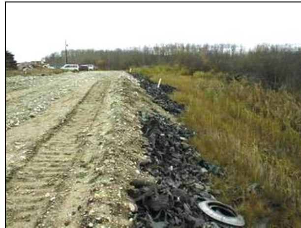
Fig 3. Tire road embankment during construction
